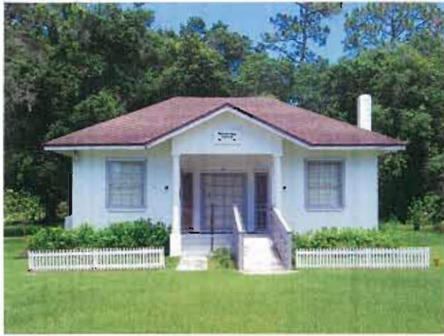
1: West Elevation - Principal Facade
