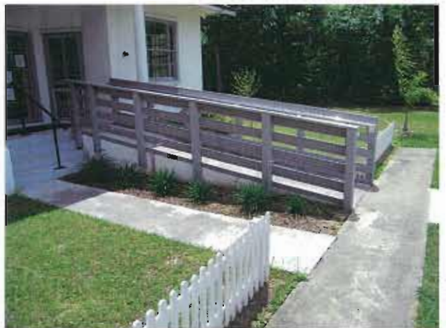
6: Accessibility Ramp at Front Entry
